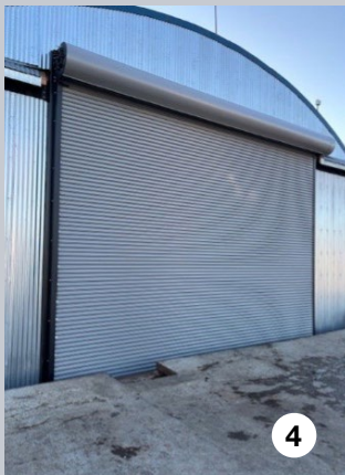
Photo 1: View from inside the boat house showing the newly installed roll-up door. Photo 2: The huge work barge shown here was needed to provide a stable base. Photos 3 and 5: A stable barge, a man lift, a fork lift, and skilled workers were all needed to remove the old sliding door. Photo 4: The new electric roll-up door is a much-needed upgrade.
